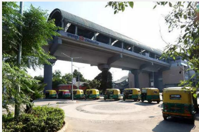
Organized IPT System, Chhatarpur Metro Station, New Delhi
